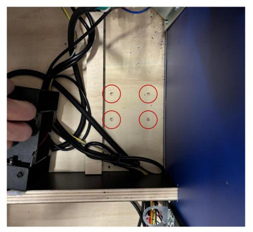
Step 2: Install shaker motor in the correct position using the 4 nut and bolts included in the kit.
